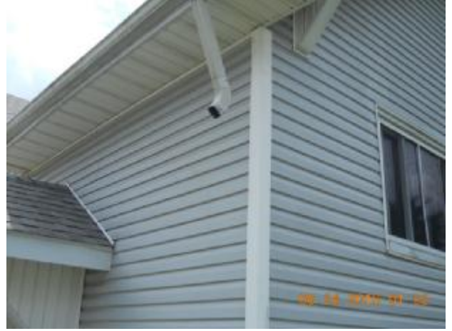
Missing downspout
