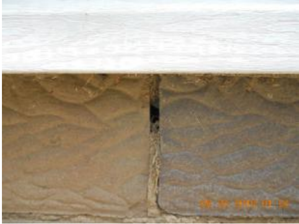
Missing mortar
