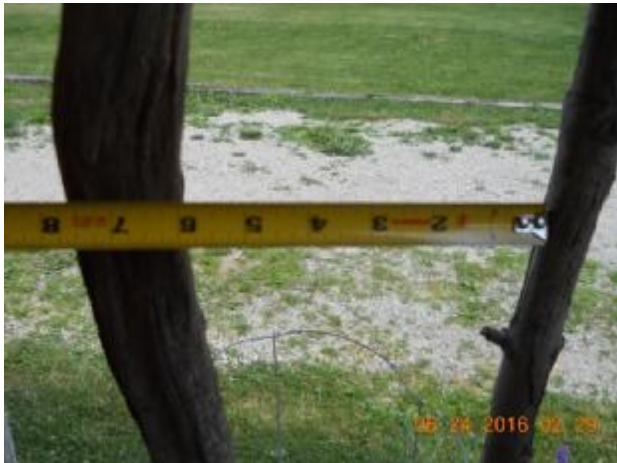
Balusters should be 4 in center to center
