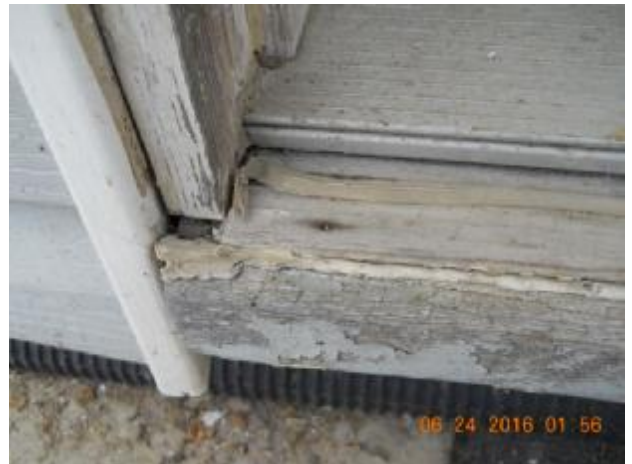
Rotten threshold
